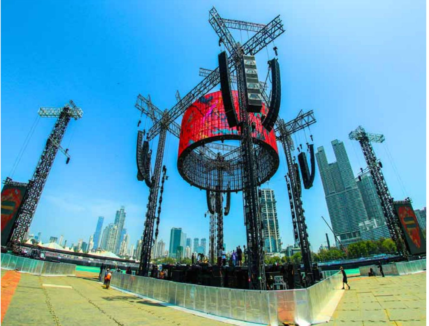
This production is a prime example of the versatility and scalability of the latest Meyer Sound technologies. The setup included 212 Panther line-array speakers in 14 arrays, 78 1100-LFC low-frequency control elements, and 22 Leopard line-array speakers. The entire Milan-based system, controlled and monitored with 26 Galileo Galaxy processors, was managed using the new Nebra software.
